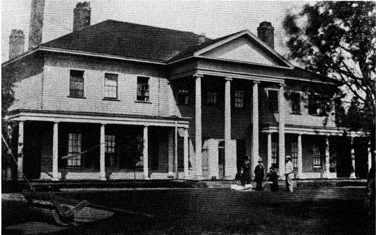
Government House built in 1834. ( Prince Edward Island Public Archives )
